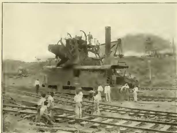
BELGIAN CANAL EXCAVATOR—CULEBRA, NEAR COLON.
